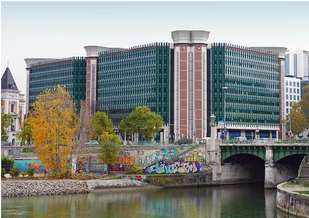
Federal Office Building Radetzkystraße, photo: BMK / Petra Grasel
